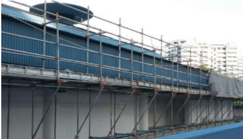
Figure 32 Cantilever Scaffold
