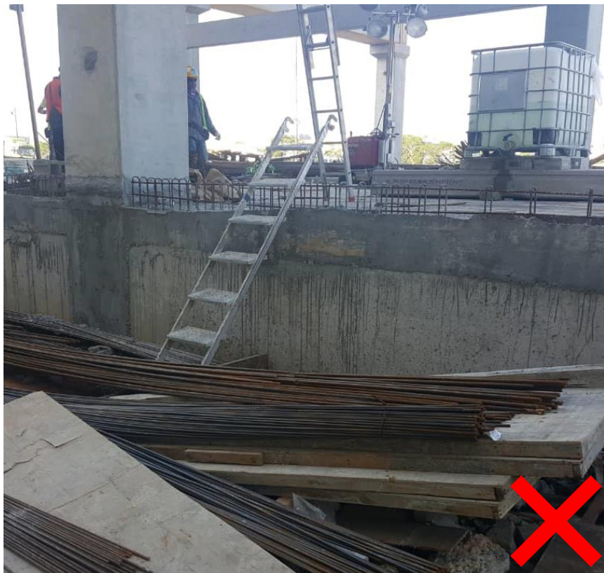
Unsafe: Scaffold and vertical ladders used to access different work areas and floors
