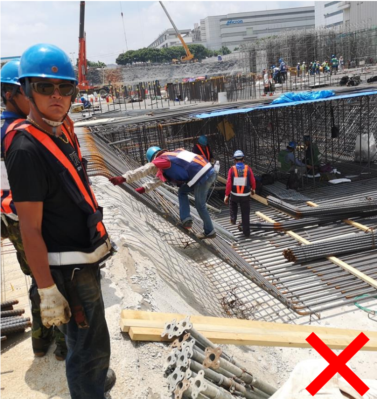
Unsafe: Workers using re-bars and timbers as alternative methods for access to work areas
