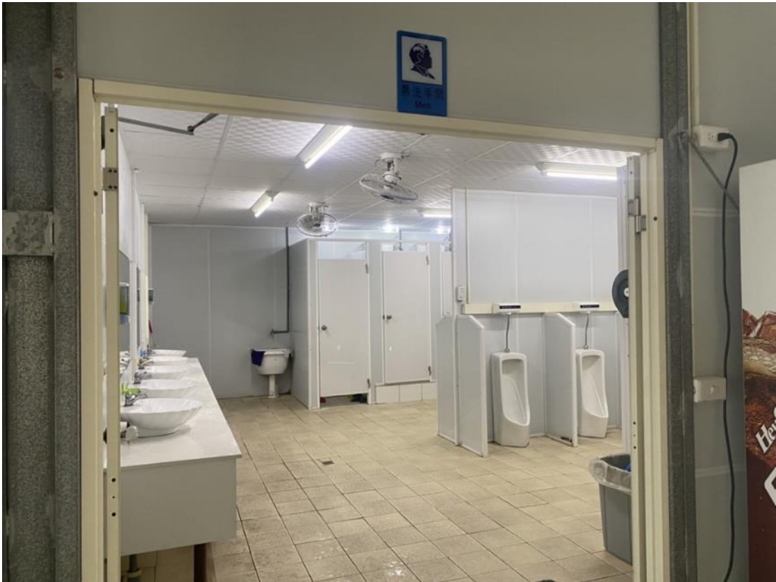
Worker toilet and washing facilities with proper temporary sanitary system including hardcore base, foundation & concrete slab finishes, toilet partition, WC, urinal & basin, prefab containerized toilet housing with fully fitted sanitary fixtures.
