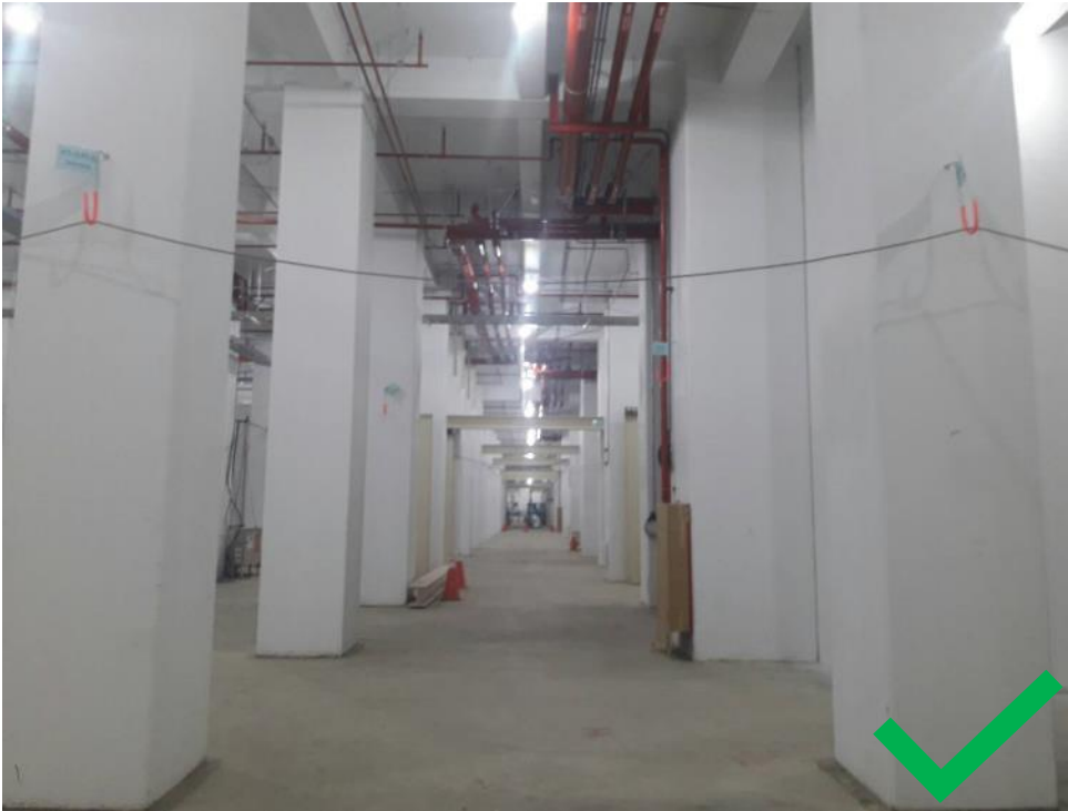
Best Practice: Electrical cables hang above 2 meters at areas used for access and egress
