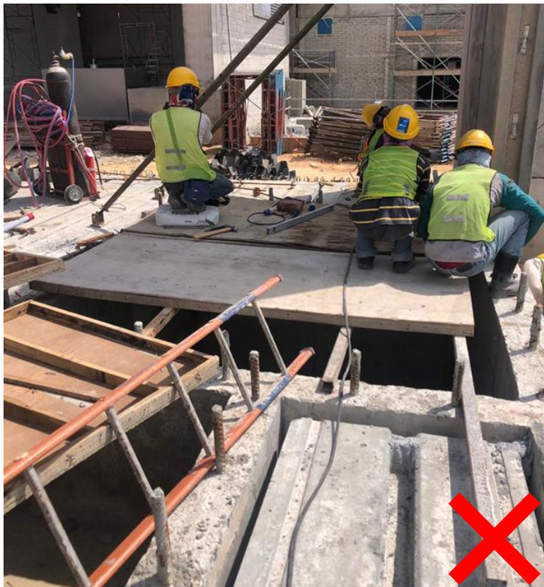
Unsafe: Hole opening covered with unsecured platform and exposed to falling hazard
